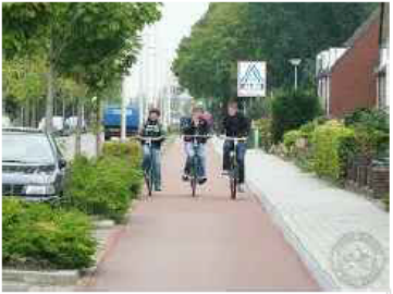
CUT INTO FOOTWAYS TO CREATE SEGREGATED CYCLE TRACK AND NARROW VEHICLE RUNNING LANES
