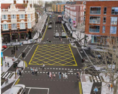
CYCLE PRIORITY THRU JUNCTION. CYCLE BY PASS, CYCLE/PEDESTRIAN ONLY PHASE AND CYCLE EARLY RELEASE
