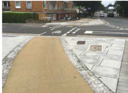
PRIORITY JUNCTION IMPROVEMENTS TO SIDE ROAD.
