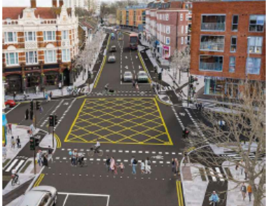
JUNCTION IMPROVEMENTS TO INCLUDE CYCLE PRIORITY FACILITIES
