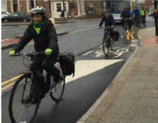
CUT INTO FOOTWAYS TO CREATE SEGREGATED CYCLE TRACK AND NARROW VEHICLE RUNNING LANES
